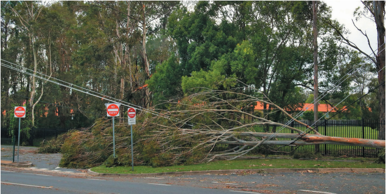
Figure 6. Powerlines damaged by fallen tree during severe storms on the Gold Coast.
