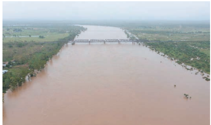
Figure 8. Flooding at Macrossan Bridge over the Burdekin River, near Charters Towers, Feb 2019
