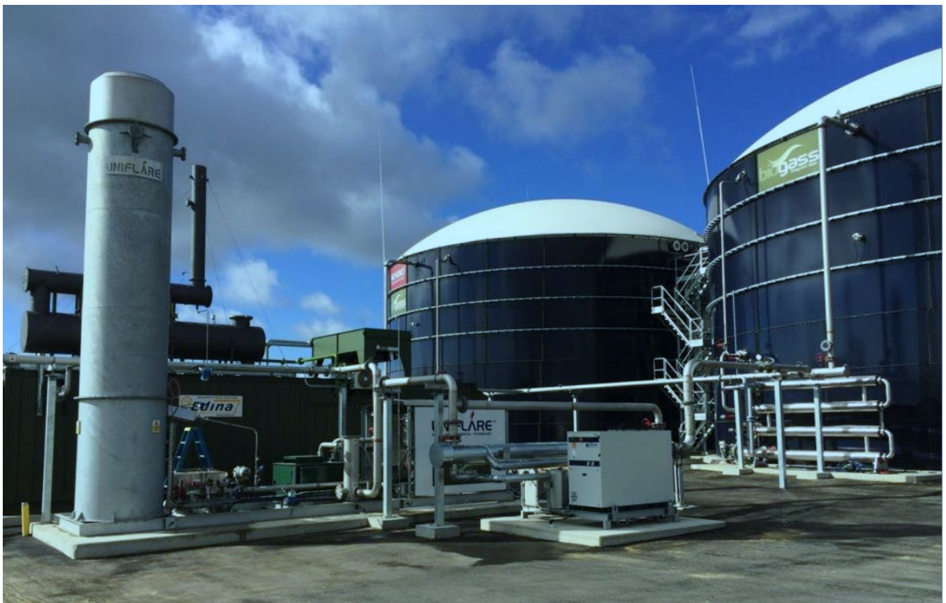
Photo 1: Richgro's anaerobic digestion facility (source: Biogas Renewables)
