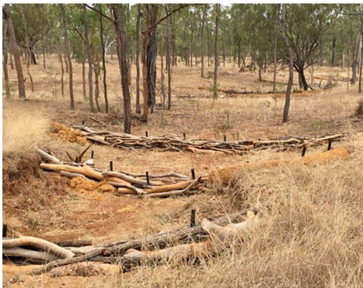
Figure 16: Using a Porous Check Dam to assist in remediating a gully.
