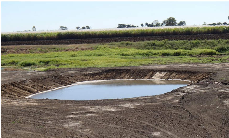
Figure 5: Top: Schematic to show how a sediment trap captures run-off water. Bottom: A newly constructed sediment trap (Source: WetlandInfo 2018e).
