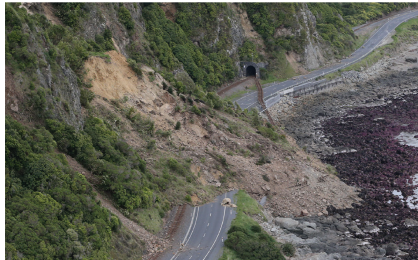
Figure 18: Impact of a landslide triggered by an earthquake in the South Island of New Zealand. Note the impact to the road and rail network. Source: Getty Images
