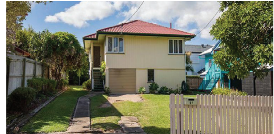
Figure 15: An example of an early post-war house. It has a Fibrolite roof that is susceptible to wind and debris damage, but its small windows make it more resilient to severe wind damage. Its timber frame makes it quite resilient to earthquake shaking. The Fibrolite roof could become a significant environmental hazard if it were damaged in an earthquake. Source: Adobe Images
