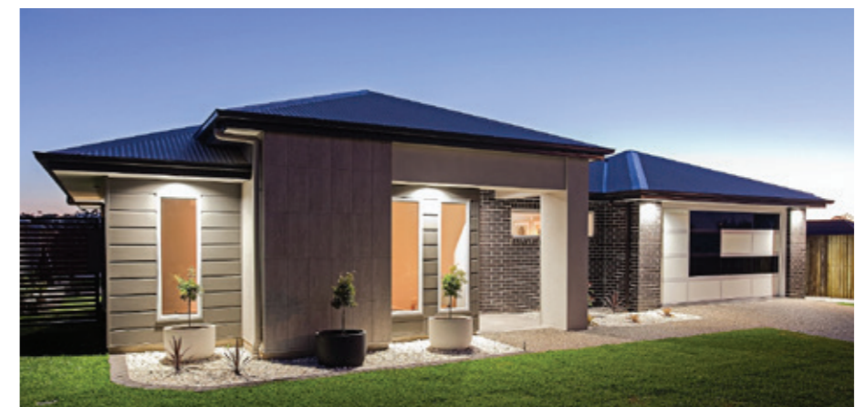
Figure 16: This is an example of a contemporary house. Their timber frames (under the brick veneer cladding) give them a degree of resilience to earthquake shaking. Source: Adobe Images
