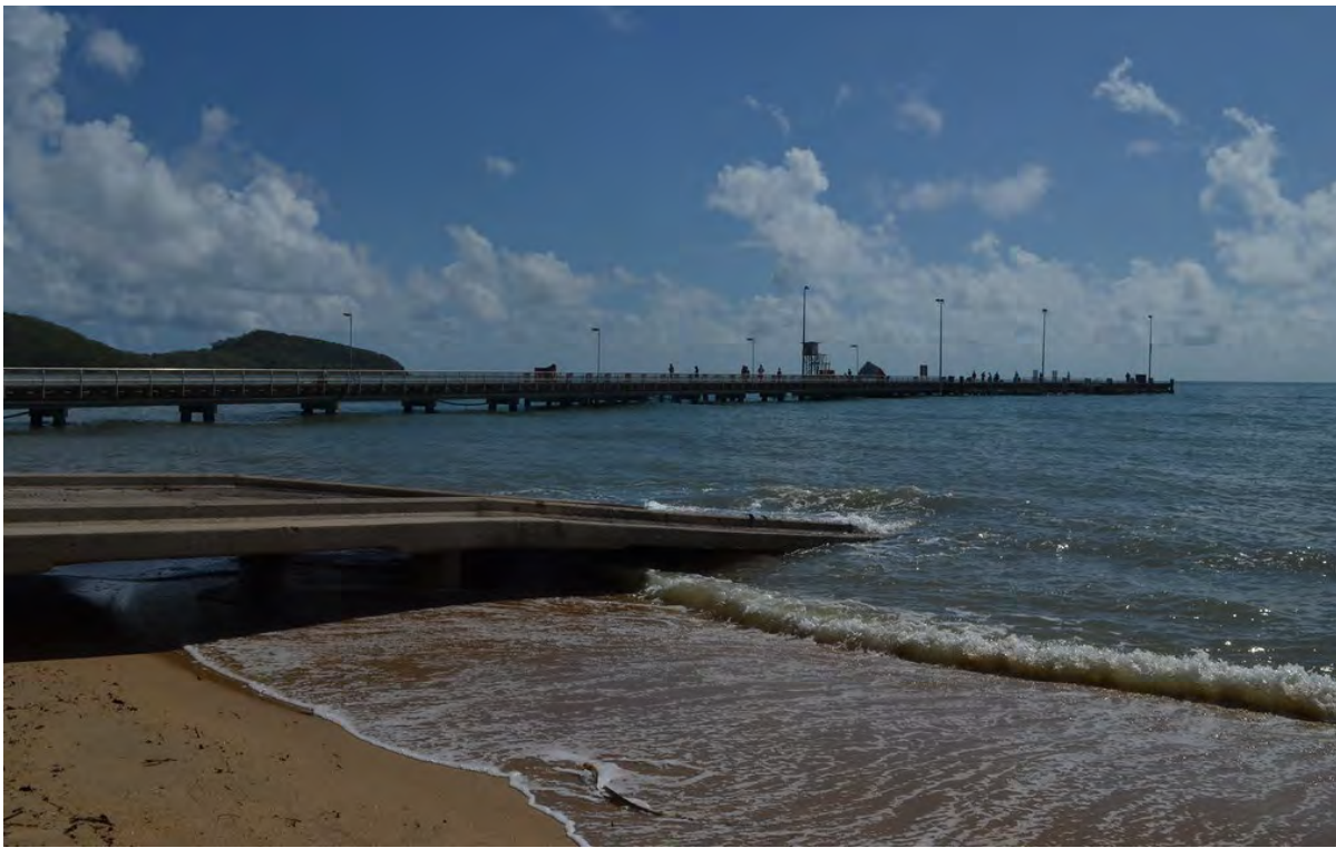
Photo 7-1 Palm Cove boat ramp (since demolished) showing elevated ramp. This is conceptually similar to what is being investigated for Sub-option 1b.
