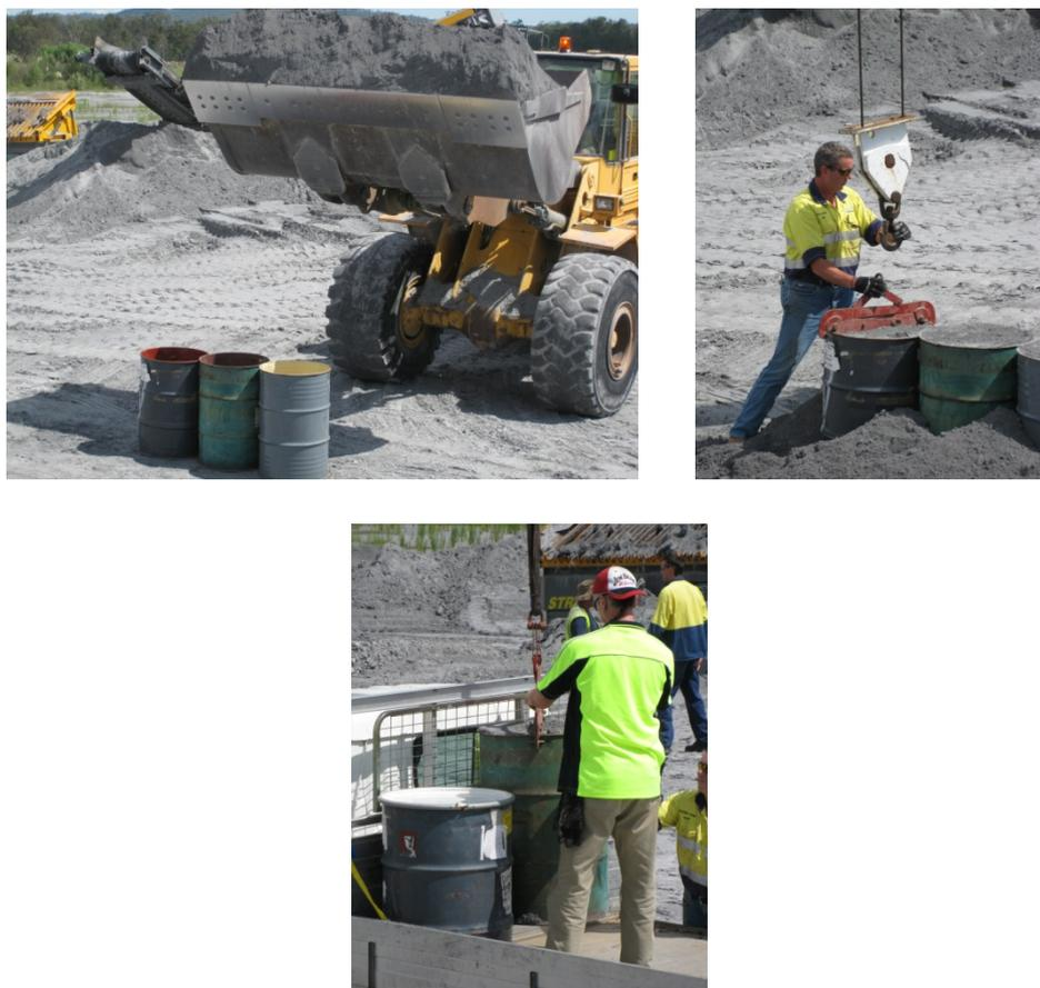
**Figure 3** Sampling Swanbank fly ash for laboratory testing
