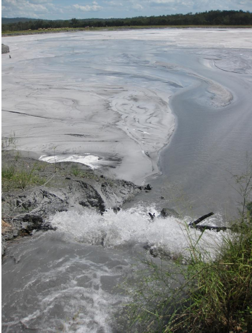
**Figure 6** A typical fly ash slurry beach at Swanbank Power Station
