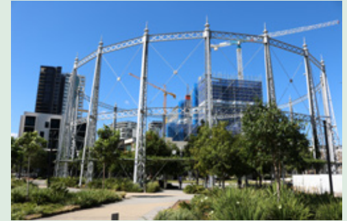
Newstead Gasworks No.2 gasholder, Newstead (QHR601594) Photo: Department of Environment and Heritage Protection
