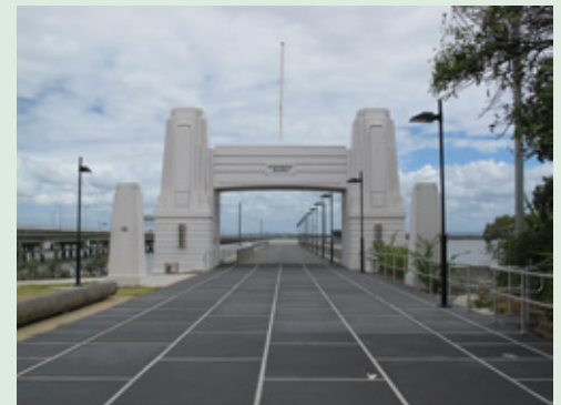
Former Hornibrook Highway Bridge Brighton (QHR 601246) Photos: Ivan McDonald Architects
