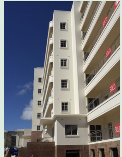
Former Townsville General Hospital, Townsville (QHR601388) Photo: CPR Townsville Holdings Pty Ltd
