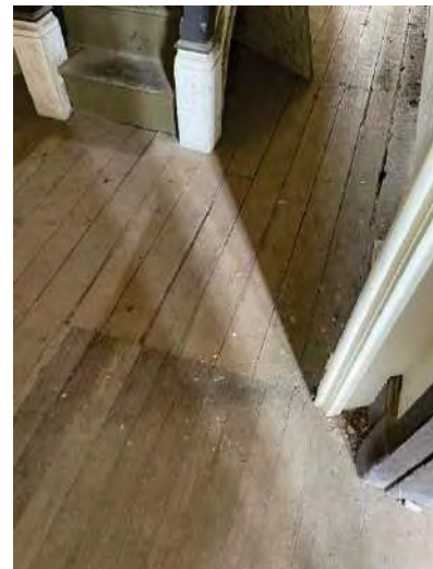
Figure 93: Photo showing patch-repair of original, thicker boards) (AHS 2021).
