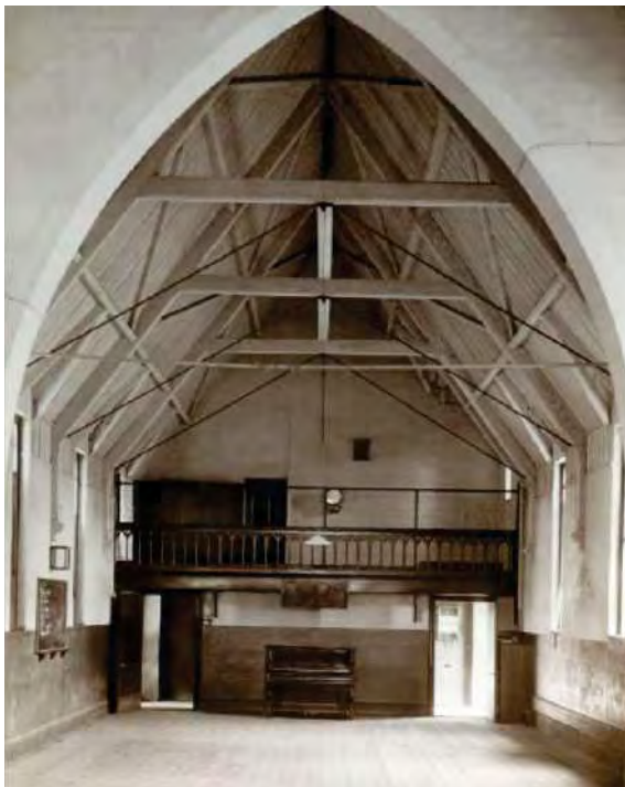
Figure 163: Great Hall, c.1929 (Ipswich Library, Reference No.: qips-2011-09-06-0009p). Note how the walls were painted, with darker colouring the lower third. Also note the door to the gallery was a four-panel door which has now been replaced (See Chapter 3 – Physical Description).
