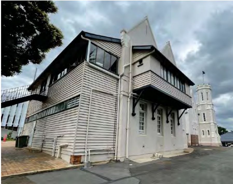
Figure 131: Bradfield House showing the southern elevation with contemporary render detail and weatherboard skillion closed verandah extension to the west. The southern façade has a matching cantilevered verandah which has been enclosed with weatherboard and FC sheeting. Note the southern tower in the background (AHS 2021).
