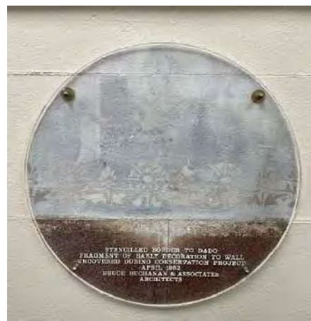
Figure 73: Detail of original paint finishes (AHS 2021).
