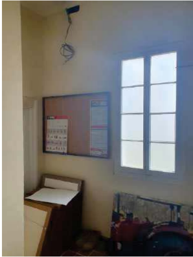
Figure 88: 1921 addition showing new room (IGS, 2022).
