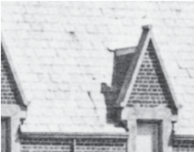
Area of roof showing slates (Detail from previous images)
