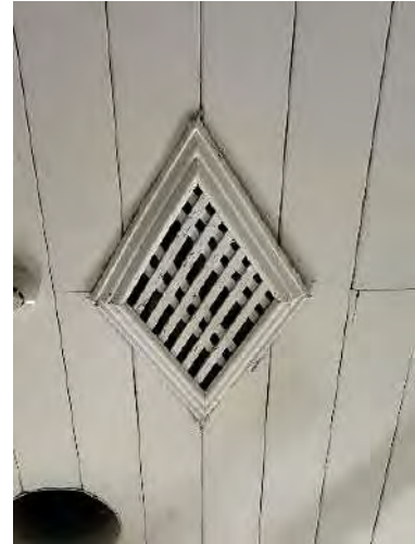
Figure 114: Diamond-shaped timber ceiling vent and flue (AHS 2021).
