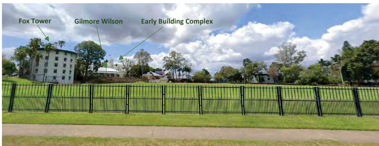
Figure 162: View from Burnett Street towards the Early Building Complex (Google Maps, 2021). Note that the bulk and scale of the Fox Tower dominates the Great Hall and Early Building Complex.
