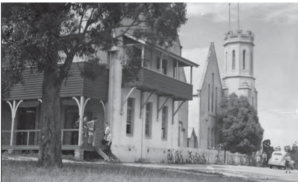
Figure 21: South West corner of the early building complex showing Bradfield House extension, n.d. (John Oxley Library, Negative No.: 202384). Note the cantilevered weatherboard balcony is not enclosed at this time and matches the detail of the northern façade addition (see Figure 19 above) (photo assumed to be c.1940s). The balcony was not enclosed until after 1965.
