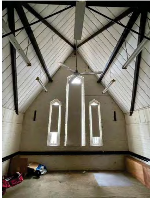
Figure 107: Room 14 facing east (AHS 2021).
