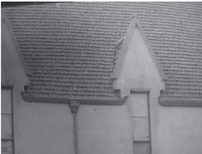
Similar area of roof showing timber shingles (Detail from previous images)
