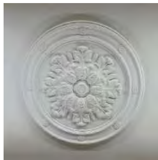
Figure 75: Ceiling plaster rose (AHS 2021).
