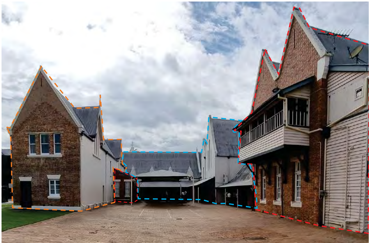
Figure 49: Image displaying courtyard area showing 1877 extensions [Orange dashed line], 1921 additions [Red dashed line], and original 1863-1865 building [Blue dashed line] (AHS 2021).
