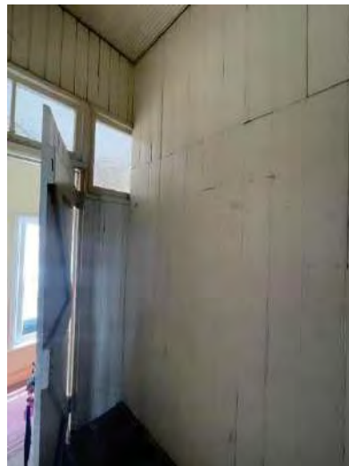
Figure 92: Wider beaded VJ wall compared to the thinner VJ (AHS 2021).
