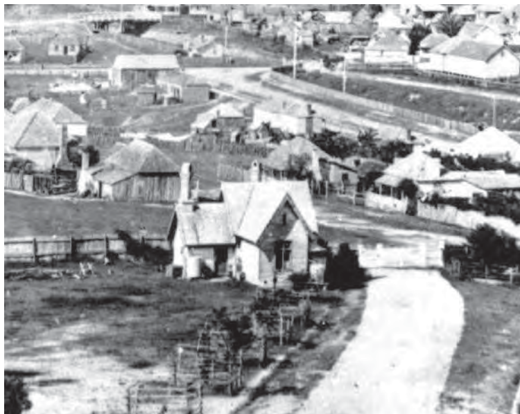
The gate keeper's cottage (Image source - Buchanan Heritage Services)
