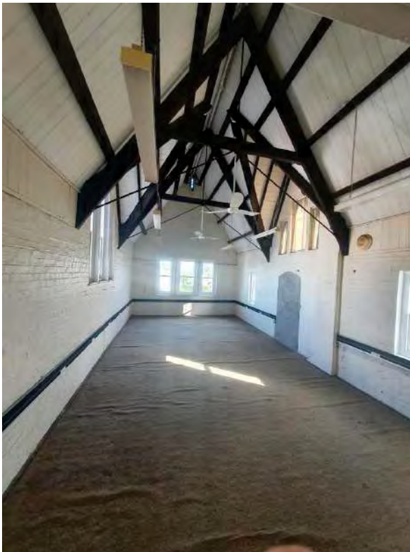
Figure 120: Room 19 facing west (IGS, 2022).
