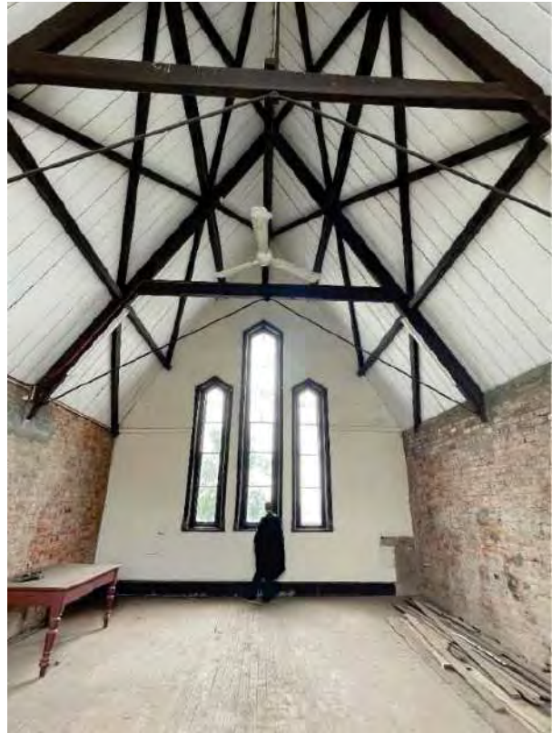
Figure 98: Room 12 facing south showing windows and exposed roof system (AHS 2021).
