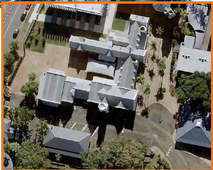
Figure 1: Study Area [blue] and the Early Building Complex including the Great Hall area, inset [orange] (Queensland Globe, 2021).
