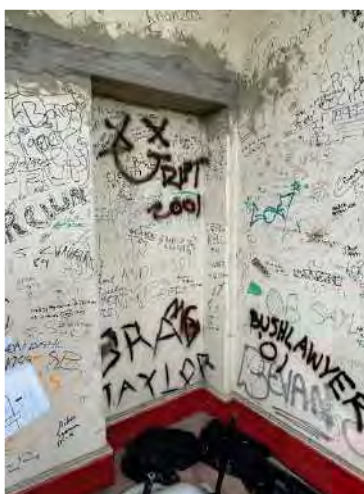
Figure 96: Room 11 showing sash windows, red-painting skirting, and original floorboards (AHS 2021).
