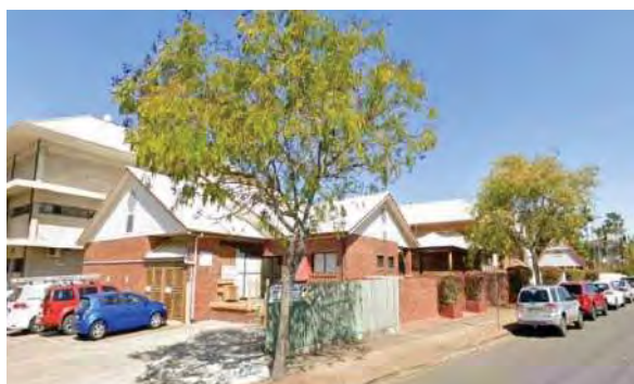
Figure 29: Street view of Woodend Road, showing the previous Murray Hancock Memorial Block and Extension prior to being demolished to facilitate the new STEM building (Google Maps, 2019).
