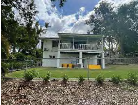
Figure 149: Boarding Master Residence (AHS 2021).
