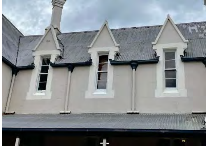
Figure 46: Dormer roofs over windows to 1863 portion of the Great Hall (AHS 2021).
