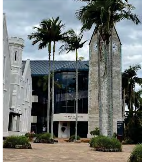
Figure 143: Entrance to the Ladley Building with Clock Tower (AHS 2021).
