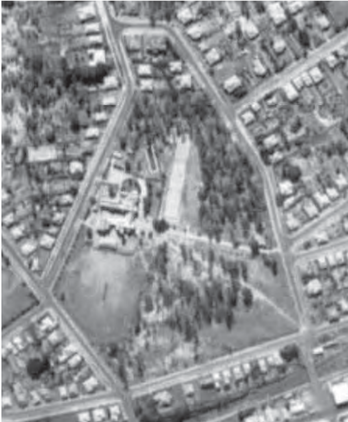
Figure 31: 1944 Aerial. Poor resolution but the original school buildings, science building and oval can be discerned. There also appears to be a strip of ground to the east of the original building which has been cleared. Note the Fig tree in the centre of the site, at what was then the top of the driveway from Waghorn Street (QImagery 2021).
