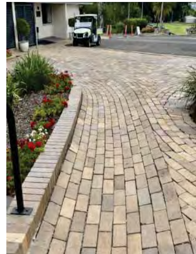
Figure 158: A low profile paved drain (AHS 2021).
