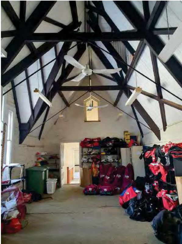
Figure 118: Room 17 facing west showing brick gable with pointed arch opening (IGS, 2022).
