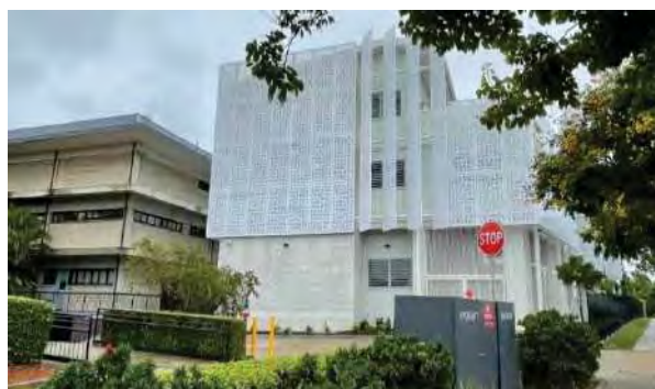
Figure 30: Street view of Woodend Road, showing the new STEM building (AHS, 2021).
