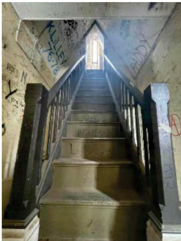
Figure 94: Narrow staircase leading up to the upper tower level (AHS 2021).
