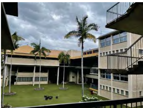
Figure 136: Clive Wyman Building and Secondary Block junction (AHS 2021).
