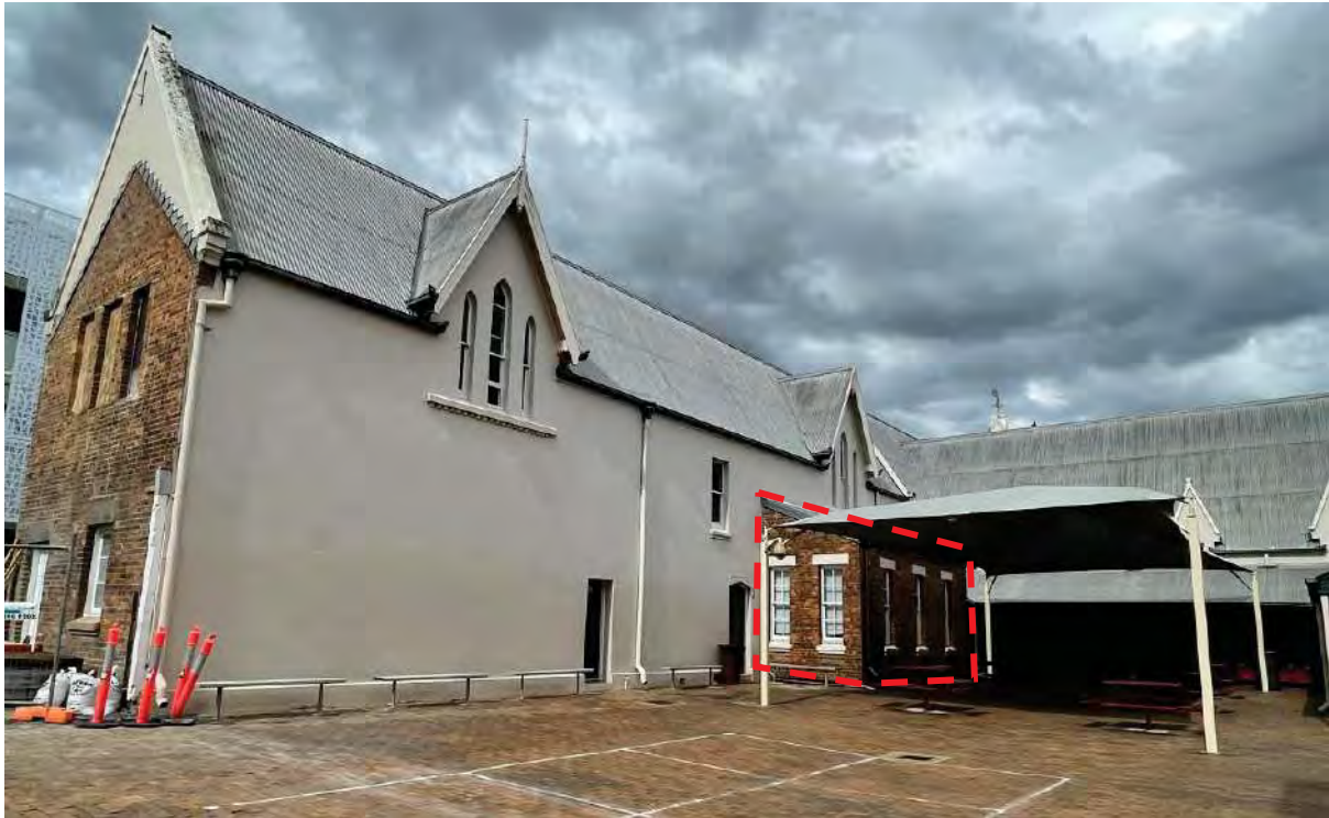
Figure 50: 1877 extension southern elevation and courtyard area. 1921 addition also indicated [Red] (AHS 2021).
