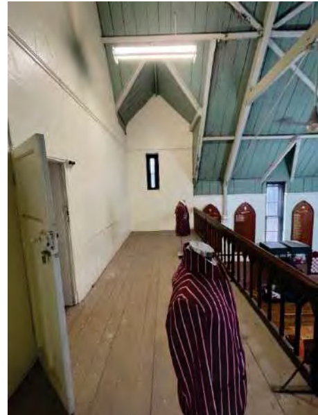
Figure 105: Great Hall Gallery showing two mannequins, original balustrading, replacement door, and a small, off-centred window to the eastern dormer (AHS 2021).
