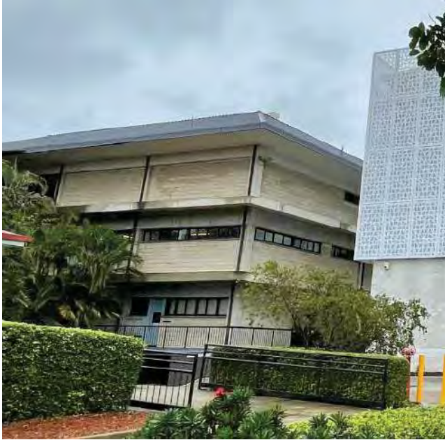
Figure 142: Rear of the Ladley Building (AHS 2021).
