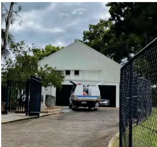
Figure 146: Headmaster Residence (AHS 2021).
