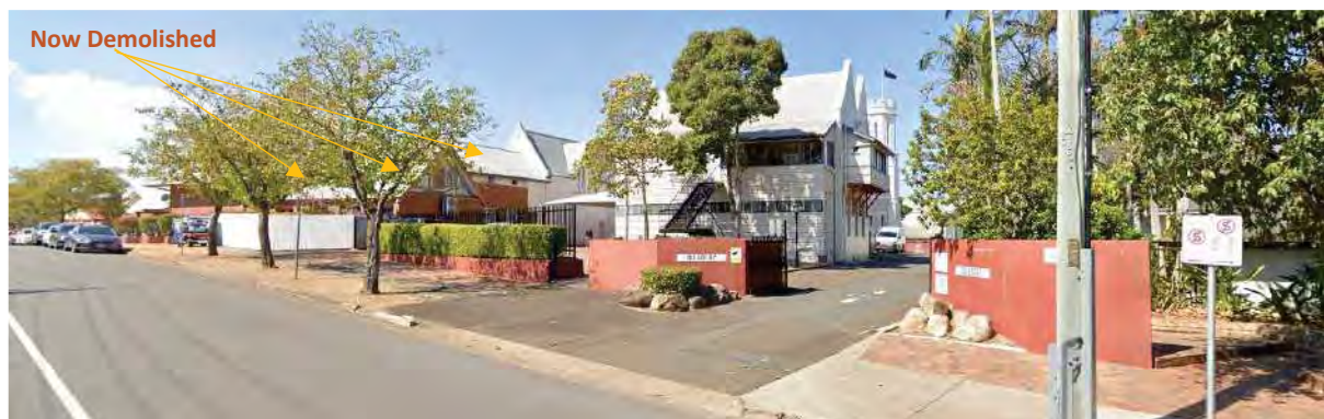
Figure 40: View of the school from Woodend Road. Note that the former dining building, accommodation and laundry building were demolished in 2019-2020 to accommodate the new STEM Building (Google Maps, 202).
