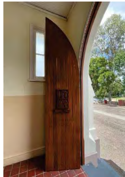
Figure 55: Arched door (side two) (AHS 2021).
