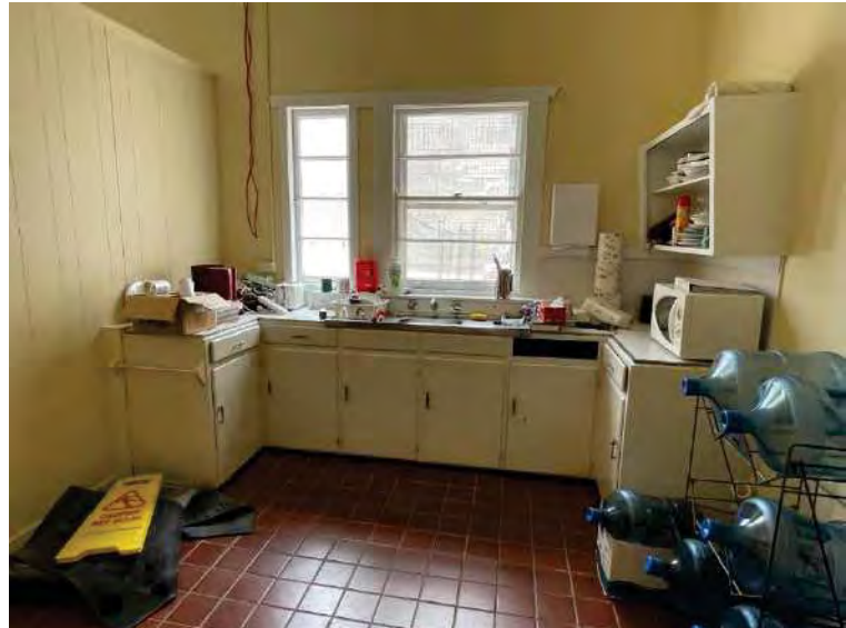
Figure 84: Room 8 kitchen area showing casement window (left window) and sash window (right window) (AHS 2021).
