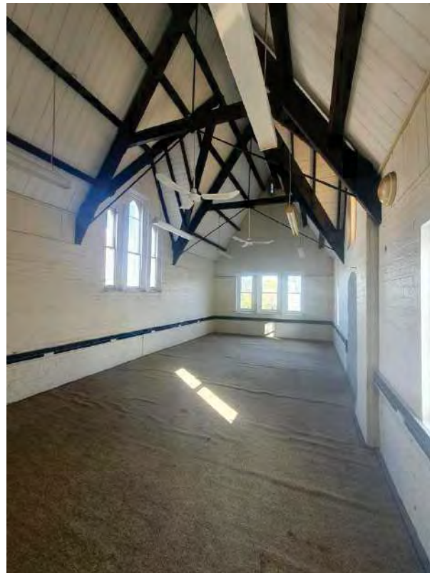
Figure 121: Room 19 facing west (IGS, 2022).
