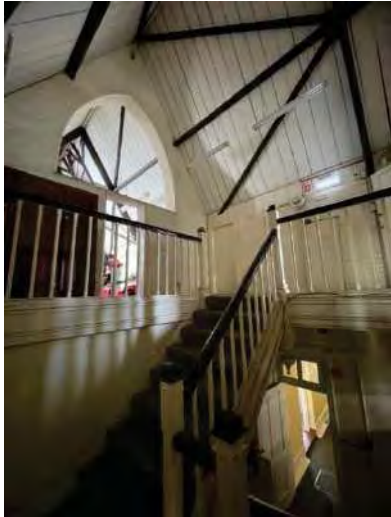
Figure 101: Stairs up to Room 13 (AHS 2021).
