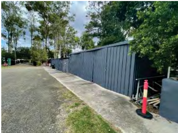
Figure 152: Garden sheds adjacent to the Hancock Oval (AHS 2021).
