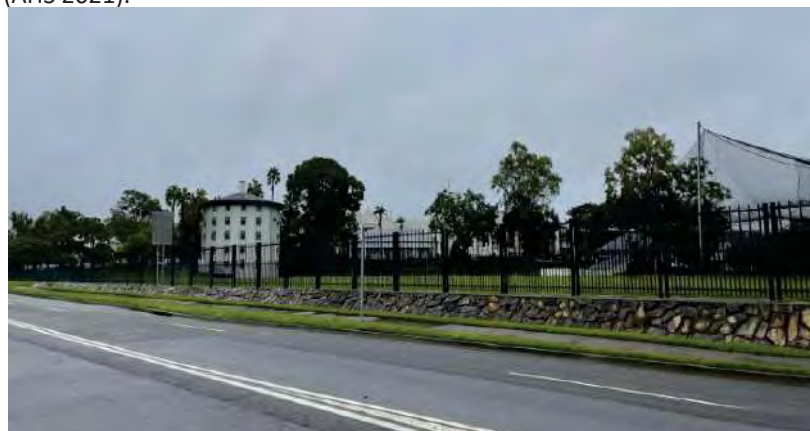
Figure 160: The powder-coated perimeter school fence and low stone retaining wall along Burnett Street (AHS 2021).
