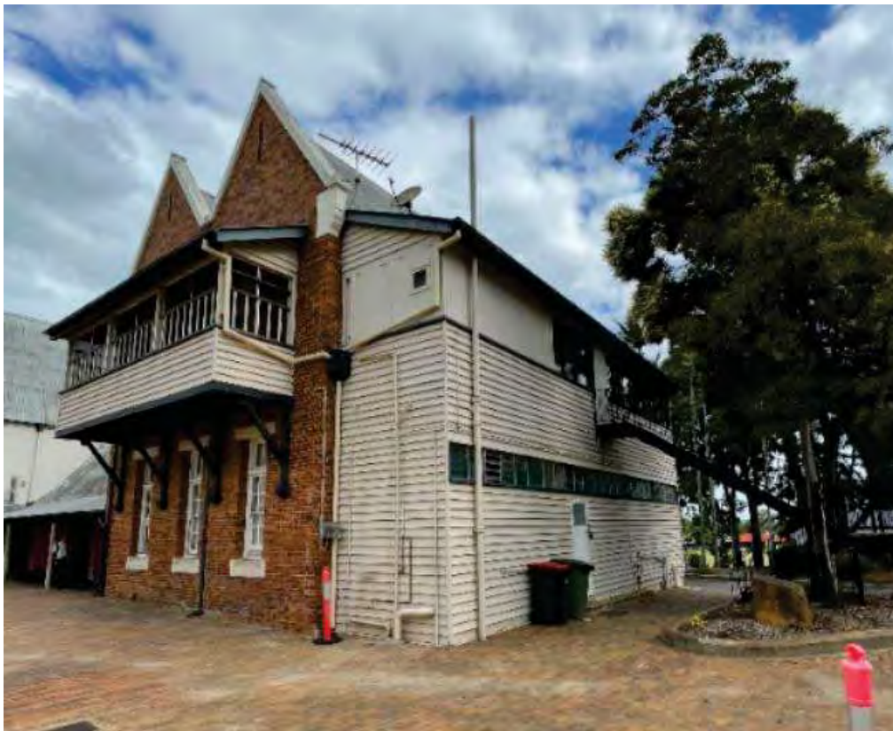
Figure 130: Bradfield House showing cantilevered room, weatherboard extension (c.1982) including external stairs, and exposed bricks (AHS 2021).
