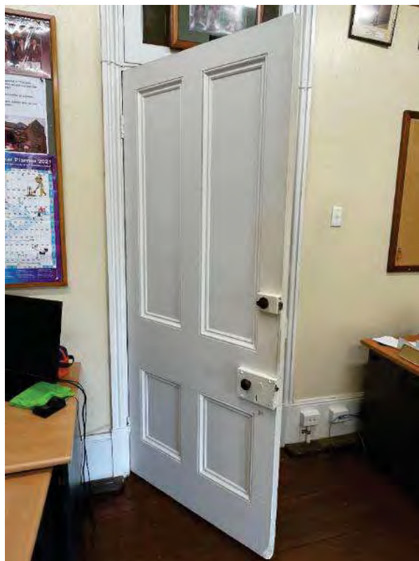
Figure 78: Original doorway to Room 6 (painted white) (AHS 2021).
