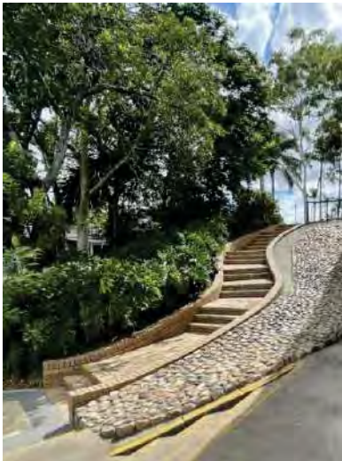
Figure 156: Brick paved walkway and stone-work set in concrete (AHS 2021).
