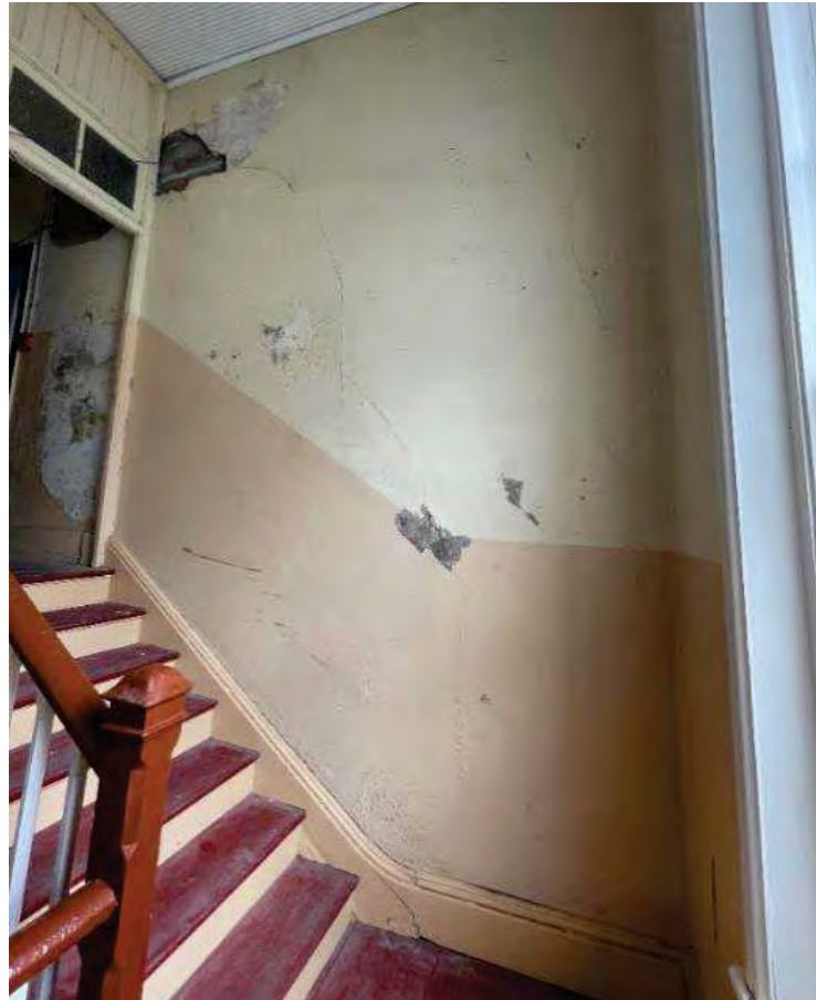
Figure 90: Staircase to the First Floor and Rooms 10, 11, and 12 (AHS 2021).
