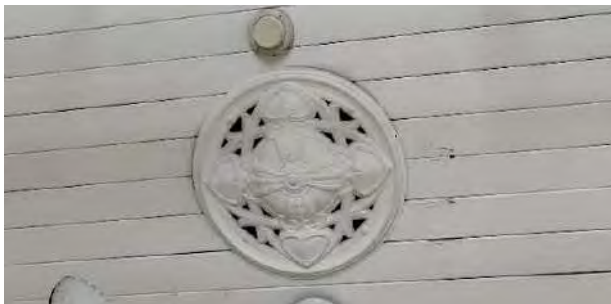
Figure 108: Room 15 early ceiling rose (AHS 2021).
