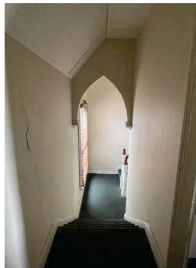
Figure 126: Small staircase from Room 16 down into Area 20. Note the pointed archway (AHS 2021).
