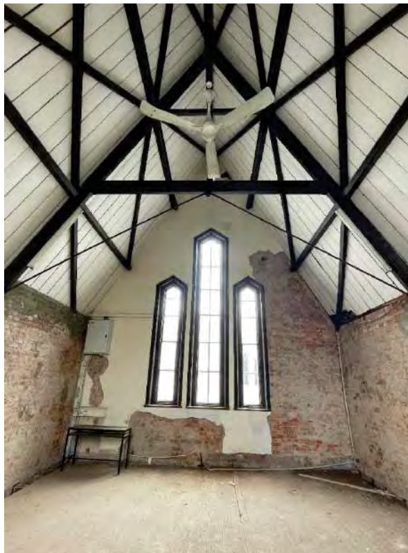
Figure 99: Room 12 facing north (AHS 2021).
