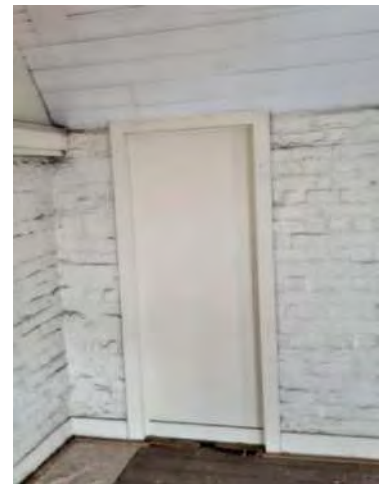
Figure 115: Enclosed doorway on southern wall (IGS, 2021).
