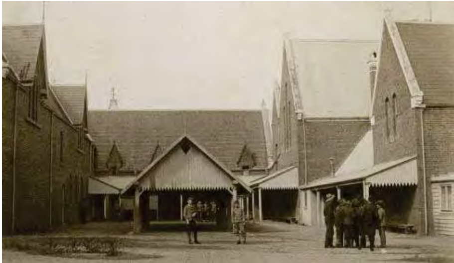
Figure 22: Quadrangle / courtyard, c.1910 (Ipswich Library, Reference No.: qips-2011-09-06-0035p). Note the small gabled structure in the centre that has long since been demolished. Also note that the buildings are un-rendered on these facades in 1910, suggesting there was different phases of rendering.
