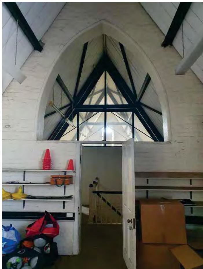
Figure 117: Brick gabled wall between Room 13 and 17 (facing east) (IGS, 2022).
