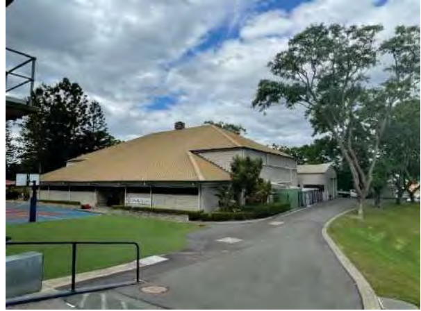
Figure 148: Photo facing Gymnasium area (AHS 2021).
