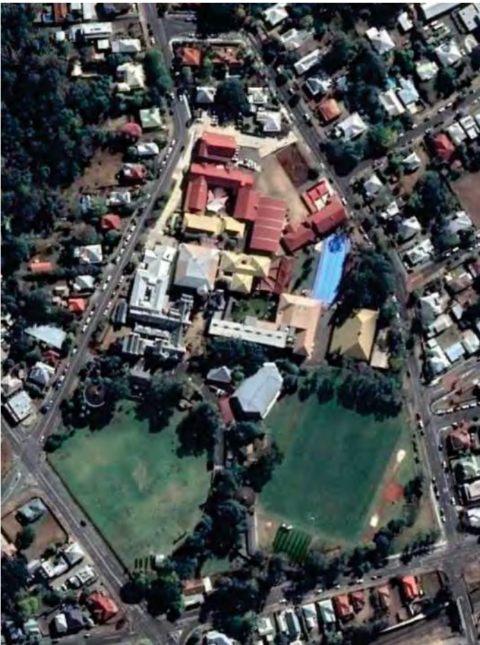
Figure 38: 2018 Aerial. One of the last aerials before the demolition of the Murray Hancock Memorial Complex (Google Earth Pro 2021).
