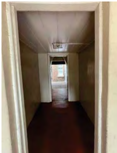
Figure 65: S.2, showing VJ ceiling (AHS 2021).
