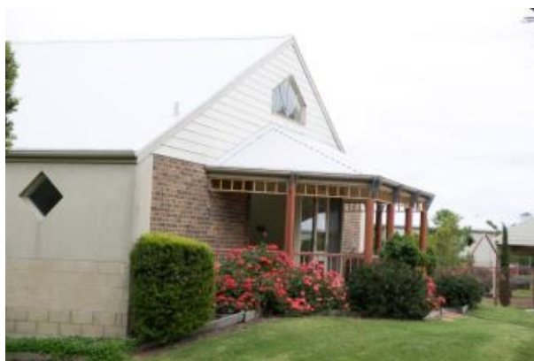
Figure 7: Reflective white paint on KRHS buildings reduces heat impacts and lowers energy demand
