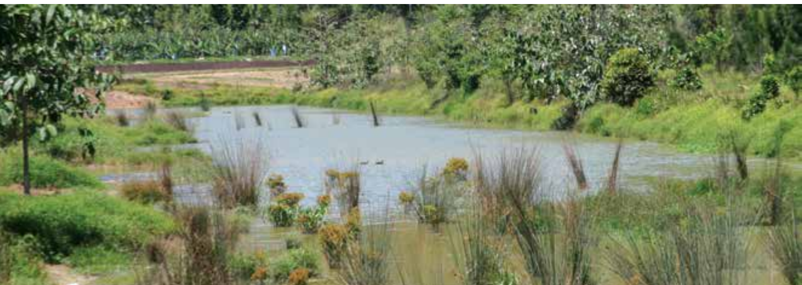
^ Constructed wetland in Innisfail—South Johnstone region
