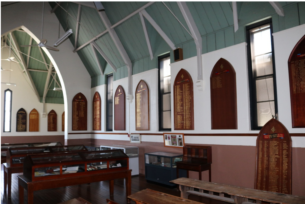
Figure 6: Main Building, school hall (Queensland Government, 2023)
