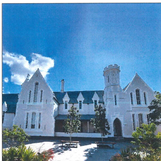
Figure 1: Ipswich Grammar School – Main Building (Queensland Government, 2023)
