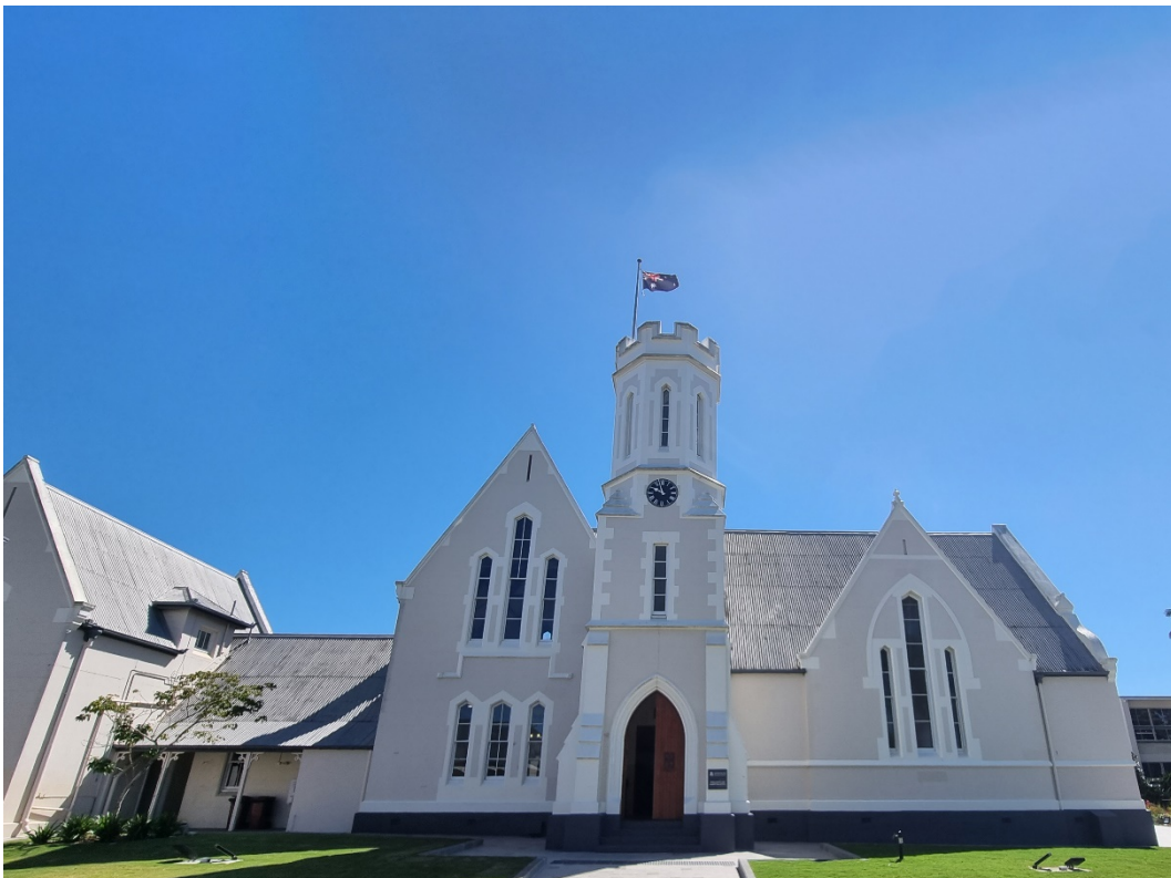
Figure 4: Main Building, 1865 Wing (Queensland Government, 2023)
