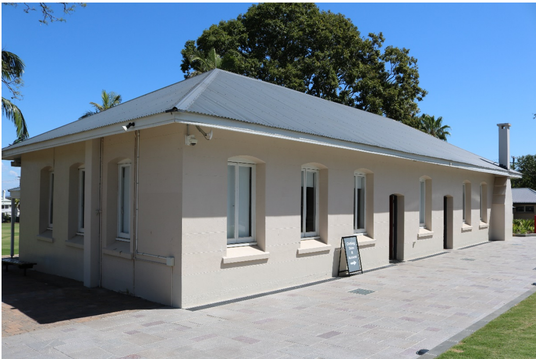
Figure 8: Science Building (Queensland Government, 2023)
