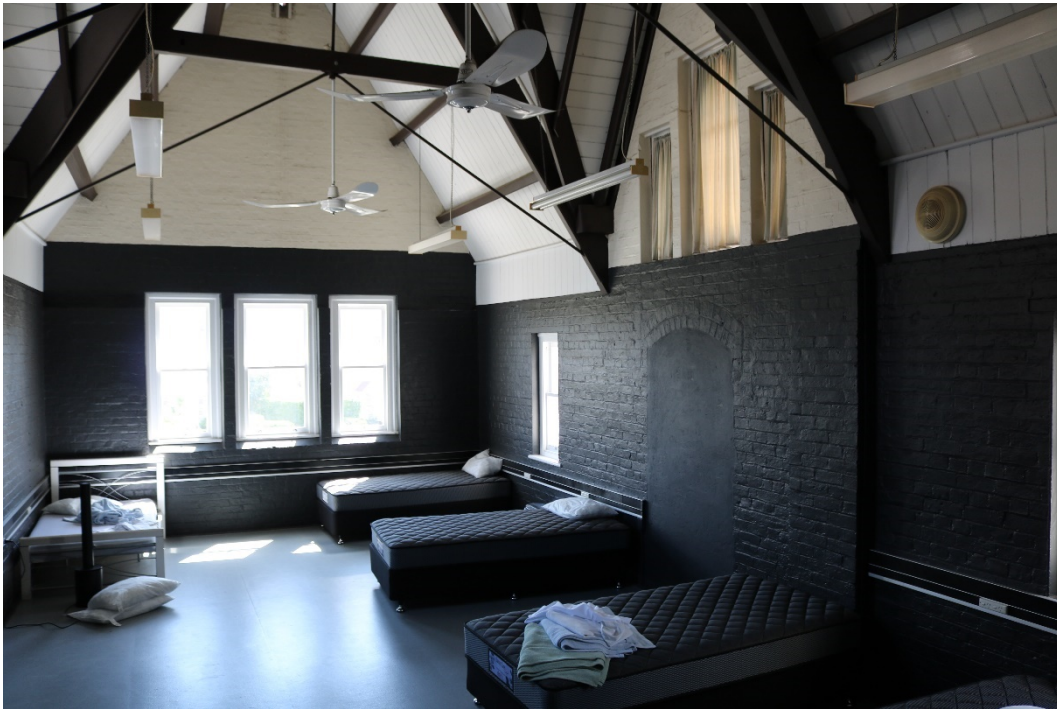
Figure 7: 1877 Wing, first floor dormitory (Queensland Government, 2023)
