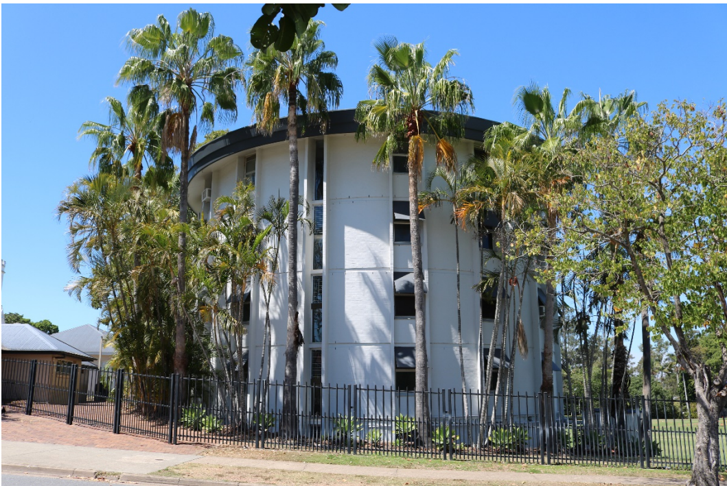
Figure 10: Fox Dormitory Tower (Queensland Government, 2023)
