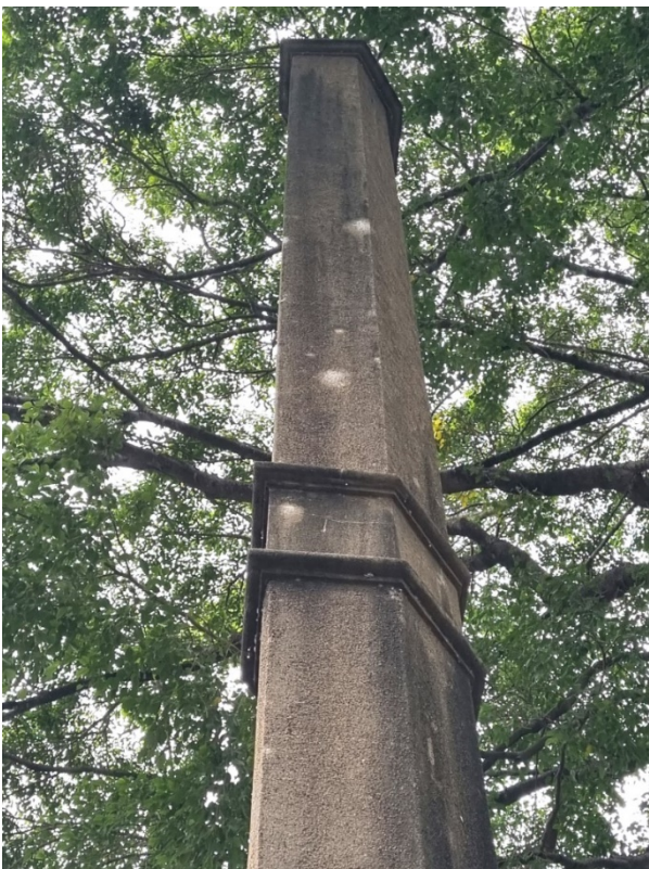
Figure 6: Vent in Parkland near Dark Street, ornamentation of shaft (Queensland Government, 2023)
