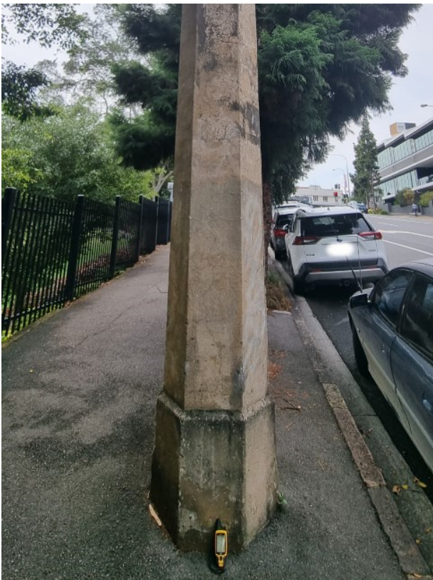
Figure 4: Vent near Twine Street, regular hexagonal base (Queensland Government, 2023)
