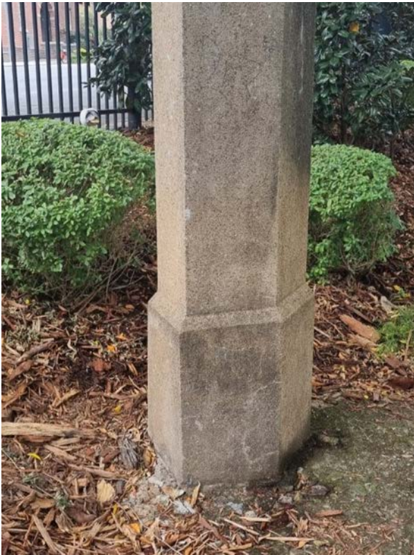
Figure 5: Vent in Parkland near Dark Street, irregular hexagonal base (Queensland Government, 2023)
