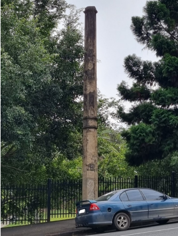
Figure 3: Vent near Twine Street, from east. (Queensland Government, 2023)
