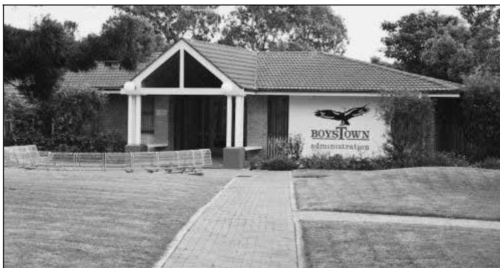
Photograph 5.10: BoysTown residential care facility (Beaudesert) (1999)—Inquiry photograph
