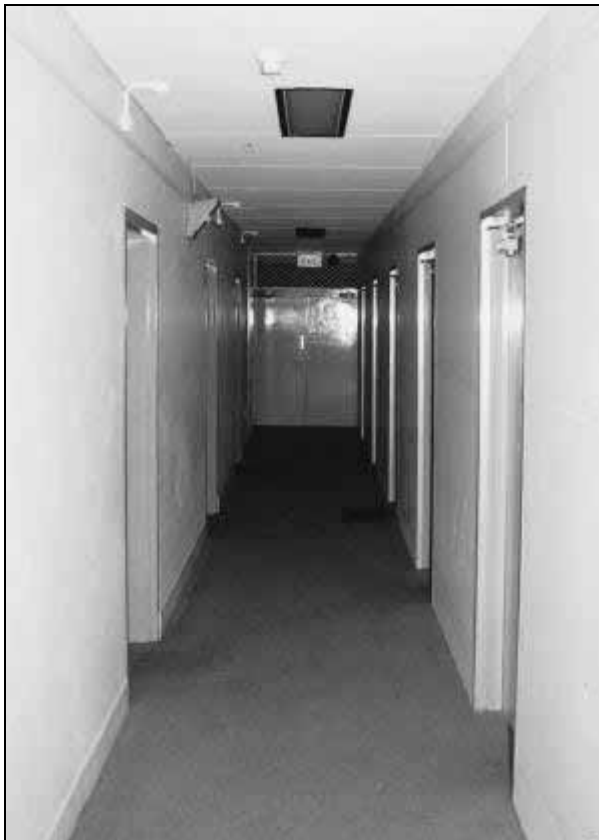
Photograph 7.13: Kalimna—dark hallway on lower level (note doorways are staggered)—Inquiry photograph
