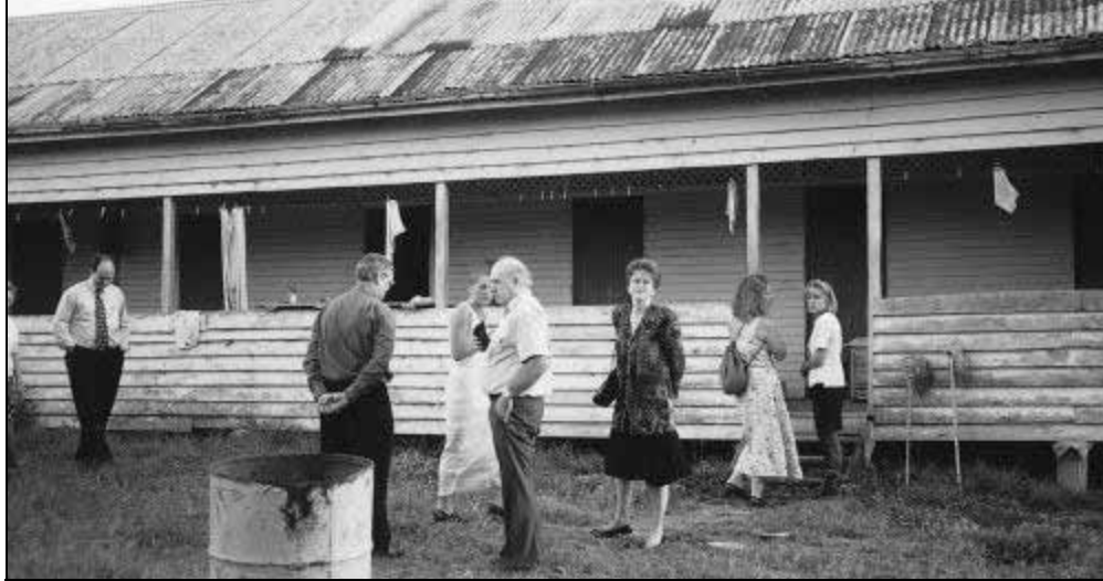
Photograph 1.1: Inquiry staff and police on site inspection—Inquiry photograph
