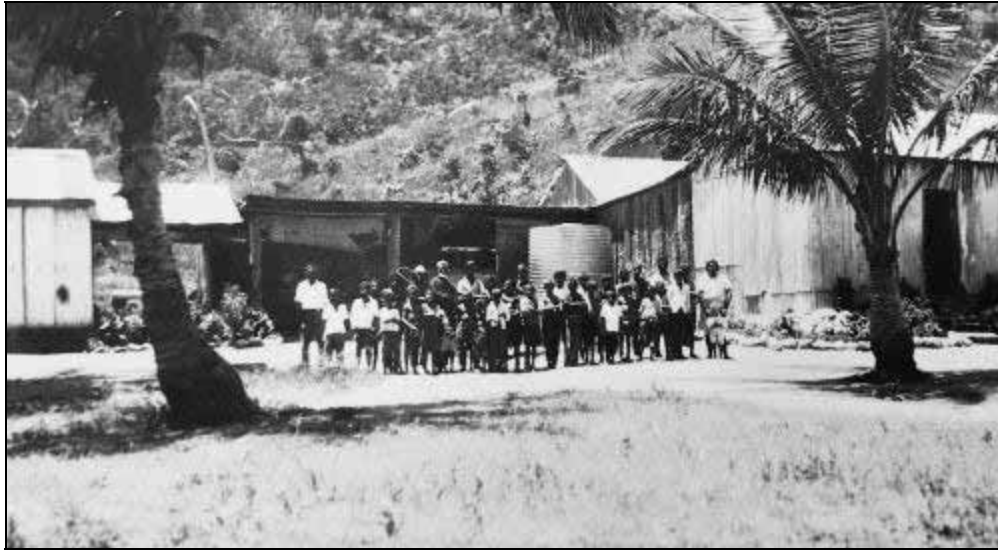
Photograph 4.3: Boys' dormitory at Palm Island (1931)—Courtesy John Oxley Library
