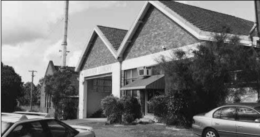
Photograph 7.14: New admissions of school age were made to work in the laundry at Mt Maria— Inquiry photograph
