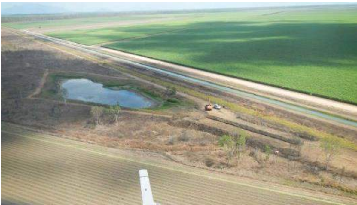
Figure 87. WetlandCare Australia sediment detention pond and constructed wetland under construction
