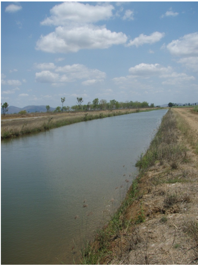
Figure 28: Reclamation sump in the Burdekin region.
