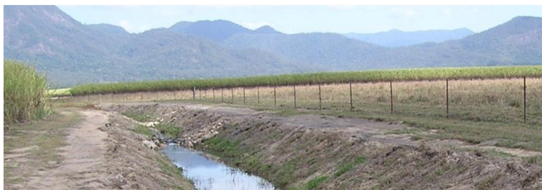
Figure 9. A constructed drain within a sugarcane field in the Tully-Murray catchment
