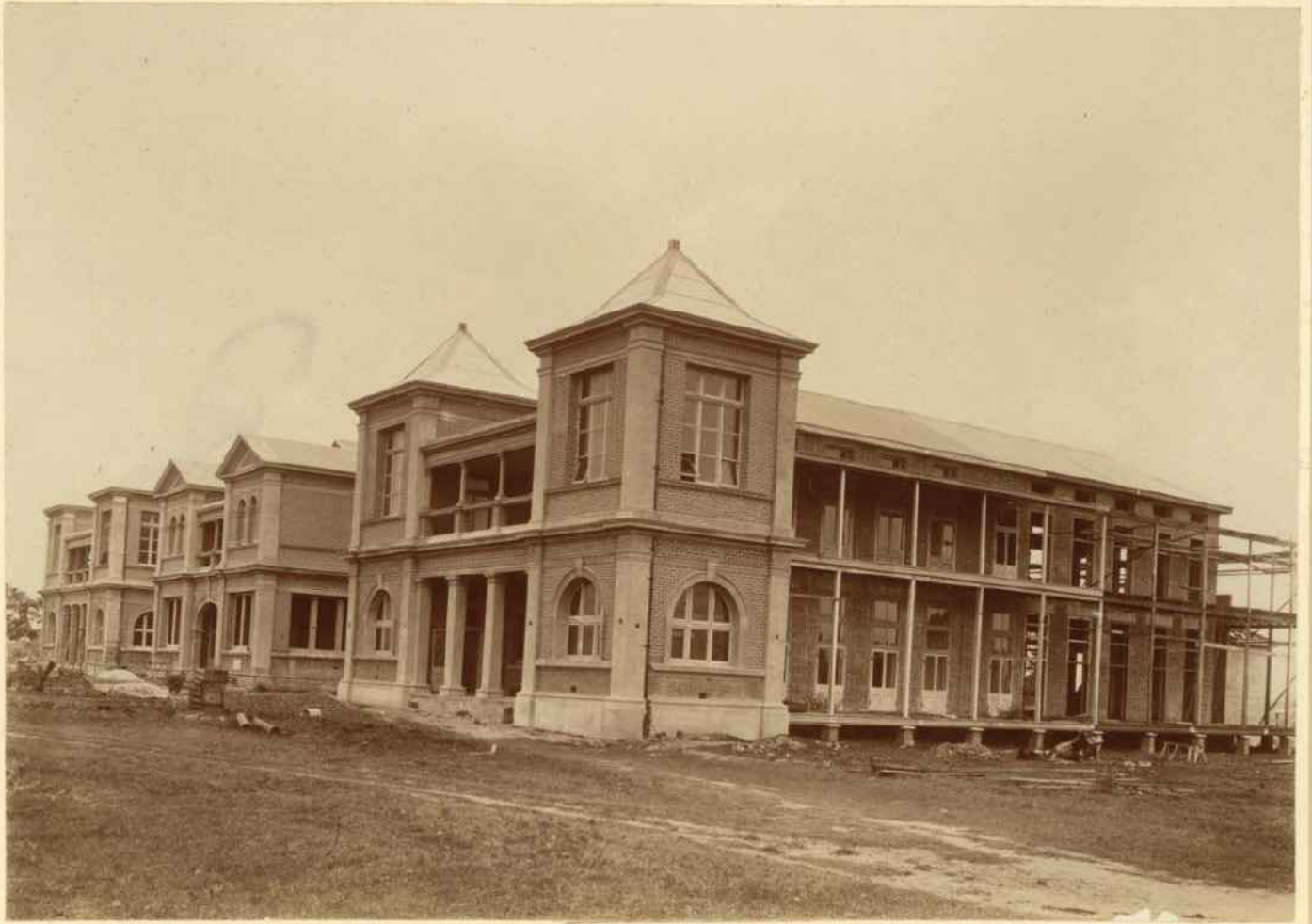
New Hospital in Course of Erection, Bundaberg.
