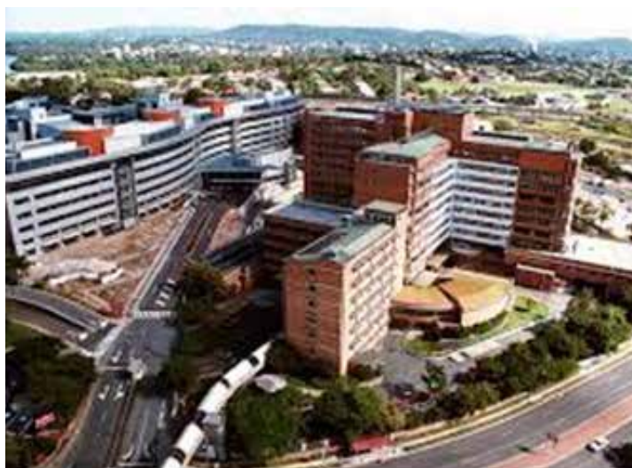
Old PAH (right) before its demolition, next to the new PAH (left)
