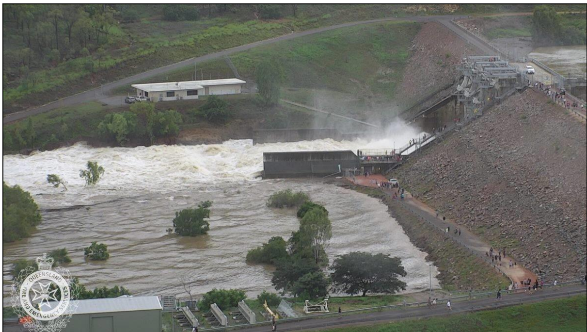
Figure 20: Image showing the Ross River Dam floodgates fully opened on 4 February 2019. Image: QFES
