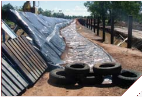
Charleville Flood Barrier
