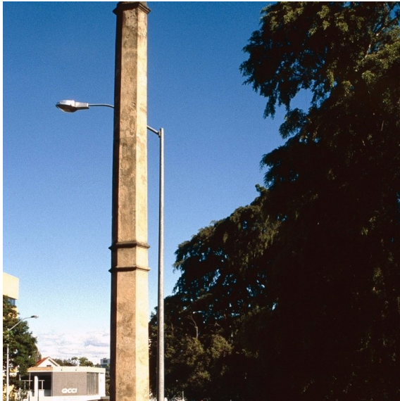
Figure 1: Monier Ventilation Shaft 1 (Spring Hill) (1998)
