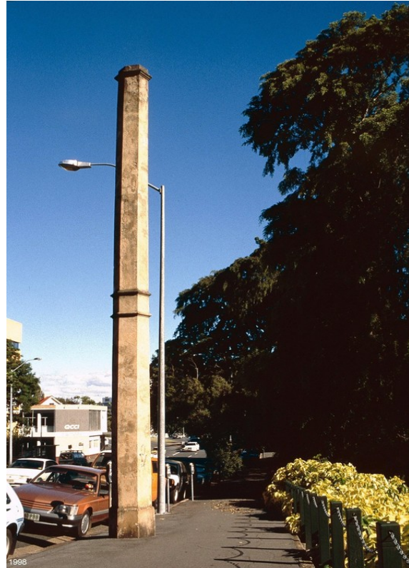
Figure 3: Monier Ventilation Shaft 1 (Spring Hill) (1998)
