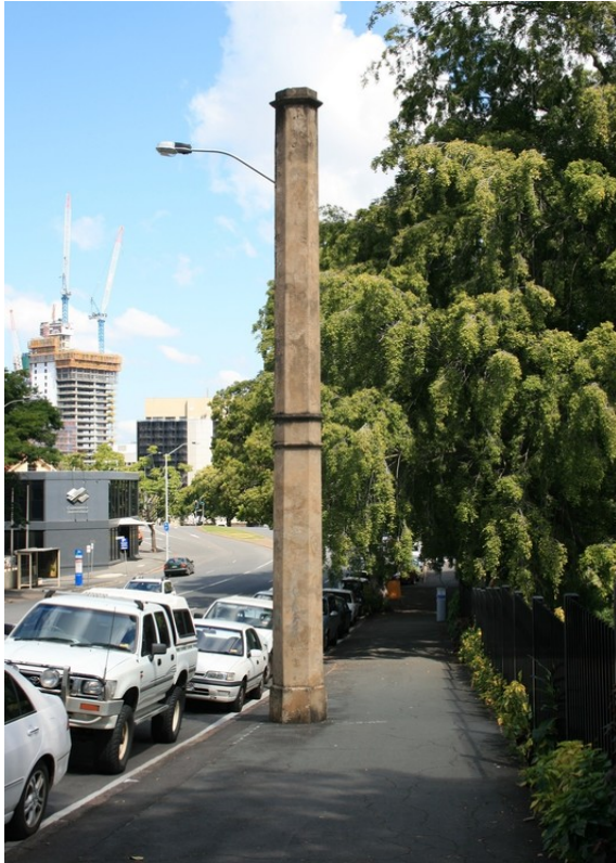
Figure 2: Monier Ventilation Shaft 1 (Spring Hill) (2008)
