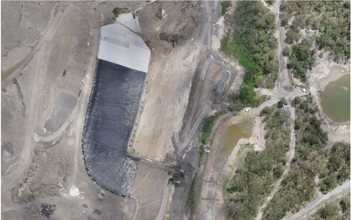
Pictured above: This photo, taken on 14 October 2022 shows the cell empty of water and the liner which will ensure any water that does enter the cell does not come into contact with waste and create odour issues.
