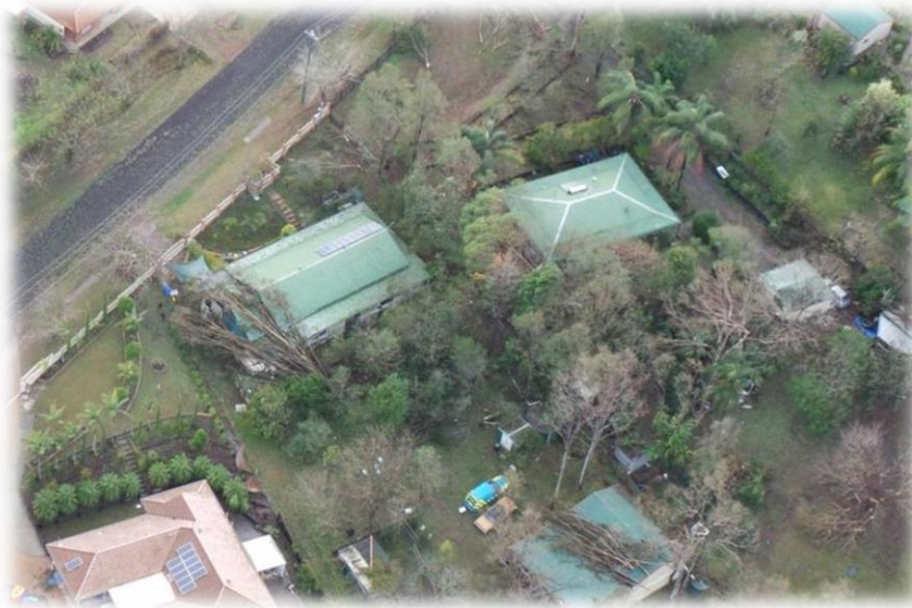
Fallen trees caused structural damage to homes in Fernvale. *Source: Twitter - penny copter
