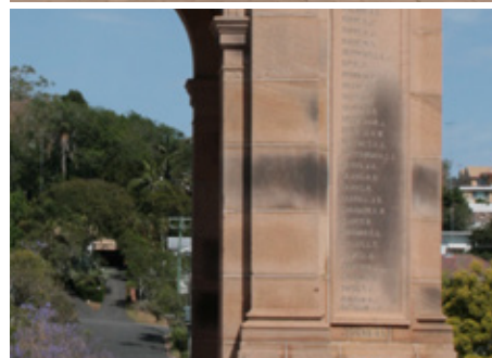
The dark patches on the Windsor Memorial [QHR 600350] are a natural oxidation of ferrous inclusions within the sandstone. While it may be possible to clean this off, it will return.
