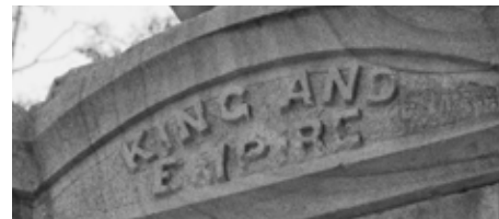
The surface of this stone appears to have been damaged by cleaning with high pressure water.
