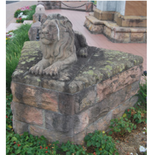
The light green patches on this stone are lichen. Bird droppings, as can be seen here on the lion's head, are a common form of staining and can cause damage.
