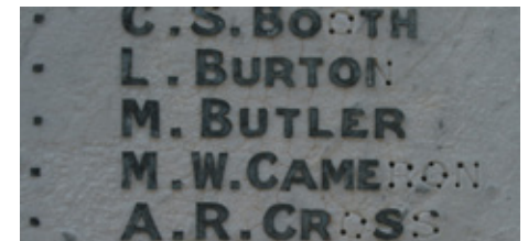
The surface of this marble has degraded and worn.
