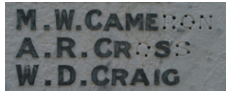
Note the holes used for fastening the missing leaded letters and the incisions outlining these letters. As these incisions wear away, the form of the lost letter will become less evident.
