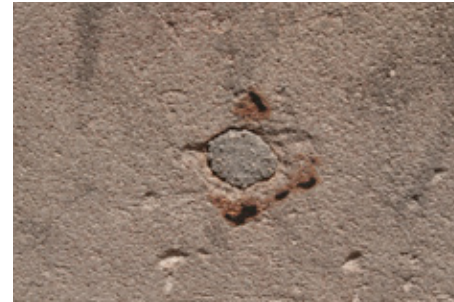
Hard cement mortars aren't suitable for repointing.
