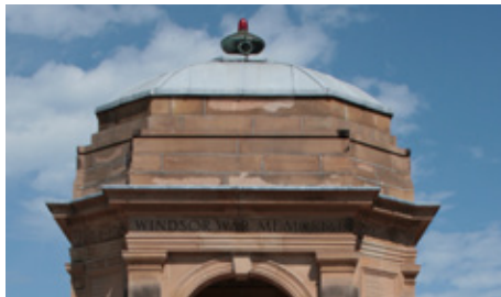
The lead sheeting on the upper surfaces of this memorial has the characteristic silver-grey patina.
