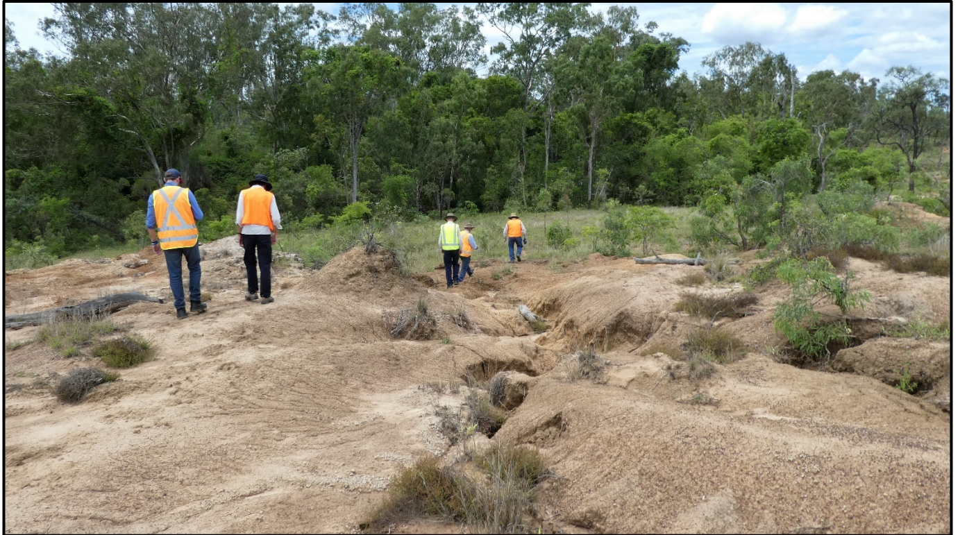
Figure 4 Deep Creek – gully erosion
