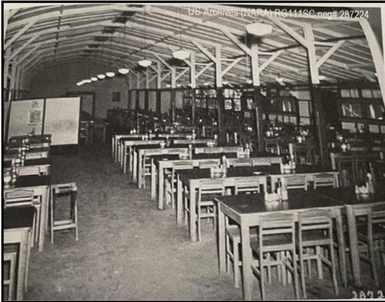
Post War, this became the UQ Vic Park Refectory. This wartime building was never intended for long term use but served varying requirements until eventual removal in the 1970s'.
