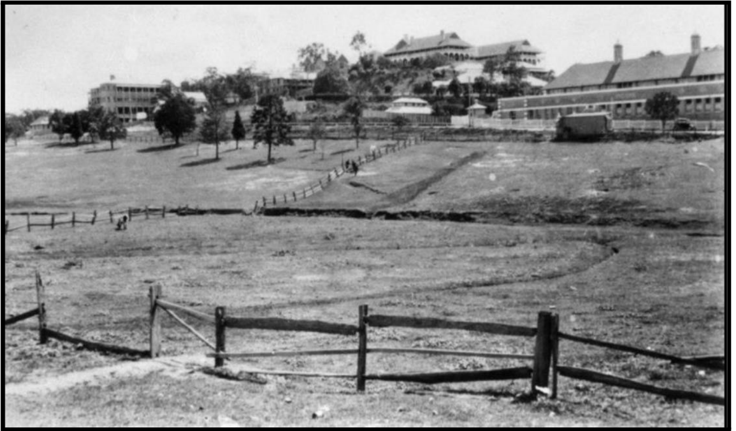
Notice that the stream which ran under Bowen Bridge Road is clearly visible in the foreground.
