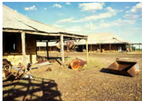
Elderslie Homestead in the Winton district in central-western Queensland contains a complex of three substantial buildings constructed from local Booka Booka sandstone in the early 1880s. It is rare in Queensland to find substantial stone buildings from this era in such a remote setting, retaining a high degree of intactness and integrity.
