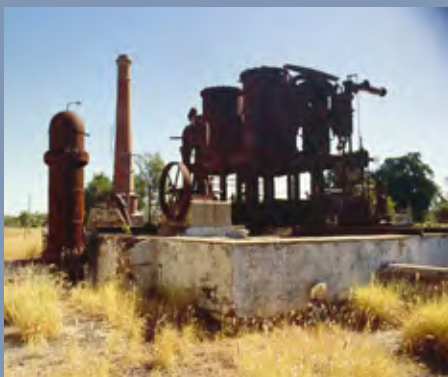
Burdekin River Pumping Station (former) (1887-1891), an archaeological site significant for its potential to reveal further information about late 19th century waterworks technology, layout, construction and materials.
