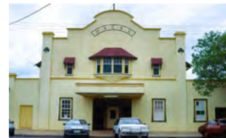
Consider the Hibernian Hall in Roma, erected in 1932 for the local branch of the Hibernian Australasian Catholic Benefit Society as a large, timber-framed hall-cum-picture theatre. The place demonstrates the characteristics of 'tropical' picture theatres, including high openings along the side walls, rows of double doors along the sides and use of lattice in the ceiling for ventilation. The place has the potential, with further study of both this and other surviving theatres, to reveal more about the nature of 'tropical' theatre design and construction during the interwar period.
