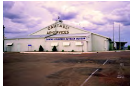
The former QANTAS Hangar at Longreach , erected in 1922 – illustrating the western Queensland origins of an important Australian and international airline.
