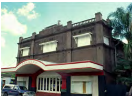
The Paragon Theatre (1927) at Childers is a rare surviving example of an interwar 'tropical' picture theatre, a once popular form of interwar picture theatre construction and design in Queensland that is no longer common.
