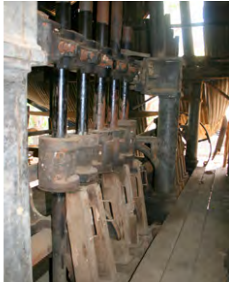
Emuford Battery (1907), Mareeba Shire, the most intact and comprehensively equipped tin battery surviving in Queensland and of rarity value for its completeness.
