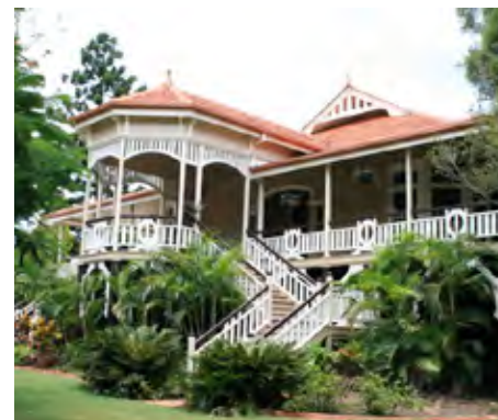
For example, JP Bottomley's House at Ipswich, designed in 1898 and constructed in 1916, is an excellent example of a substantial, decorative, high-set timber residence with wide verandahs, set within a well-maintained garden. The house now functions as the Ipswich Club .
