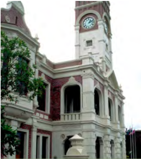
Toowoomba City Hall (1900) exemplifies this aspect of aesthetic significance. The ornately decorated street façade with its classical detailing and imposing clock tower is well composed and visually pleasing.
