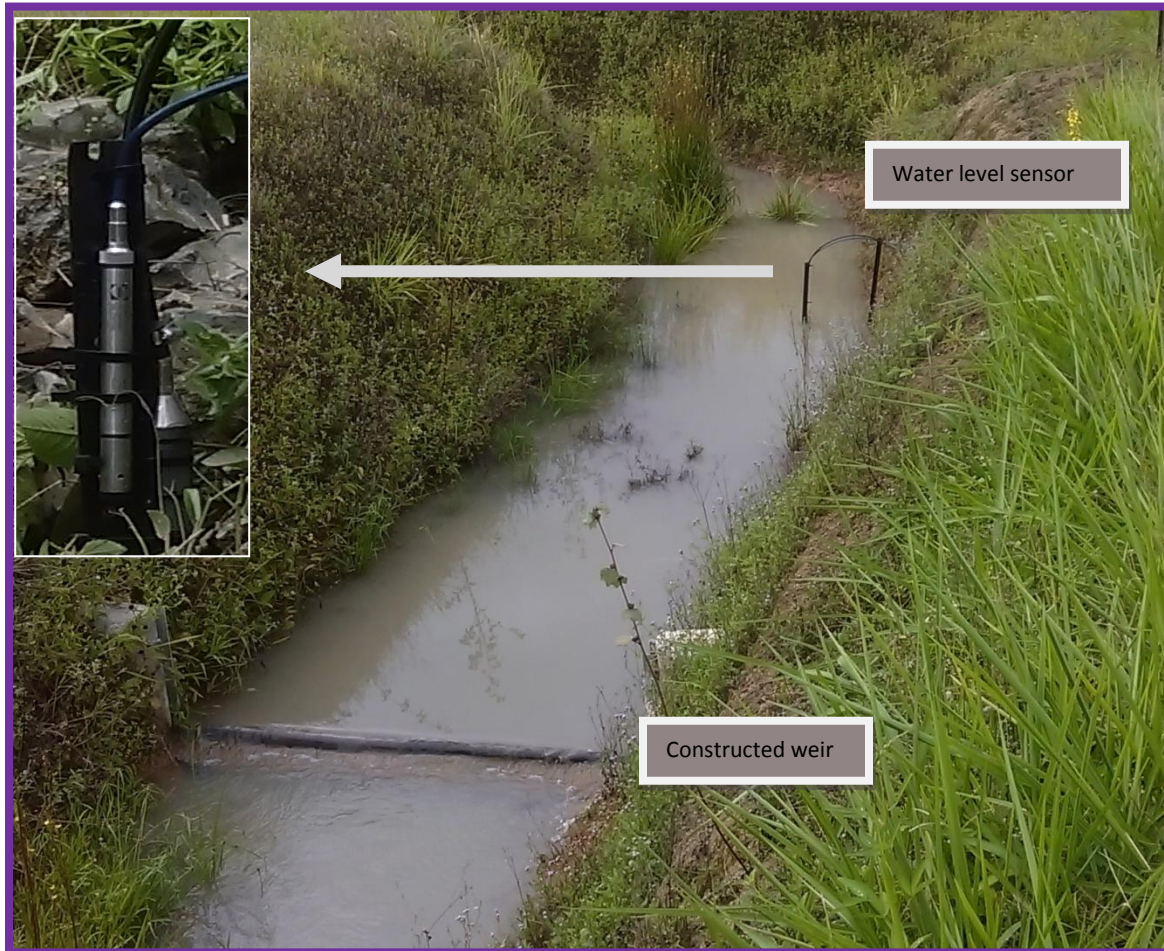
Figure 2. Weir constructed at monitoring site and water level sensor installed upstream.
