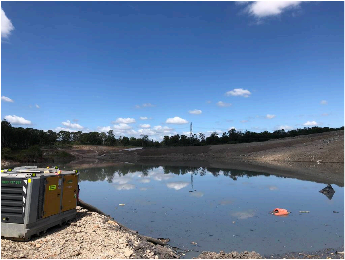
This photo from March, taken at the northern end of the cell, shows the water volume at its peak, at about 60ML.
