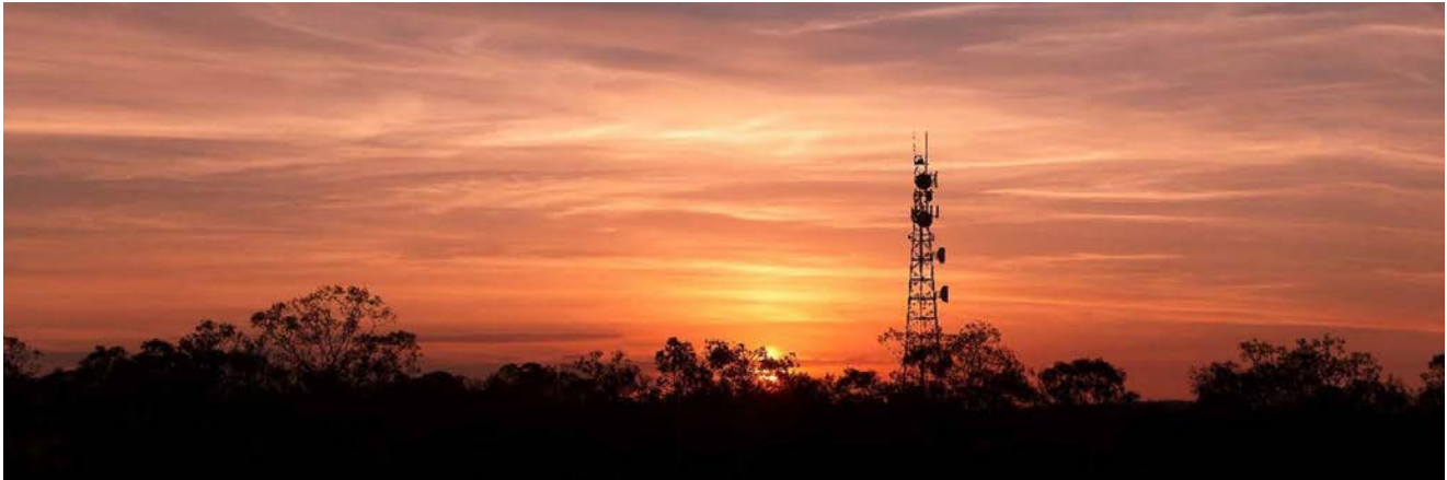
Figure 14. Communications radio tower.
