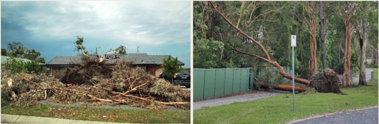
Figure 5 and 6. Gold Coast Storm Damage, 25 December 2023. Source: Cheryl van Hooft
