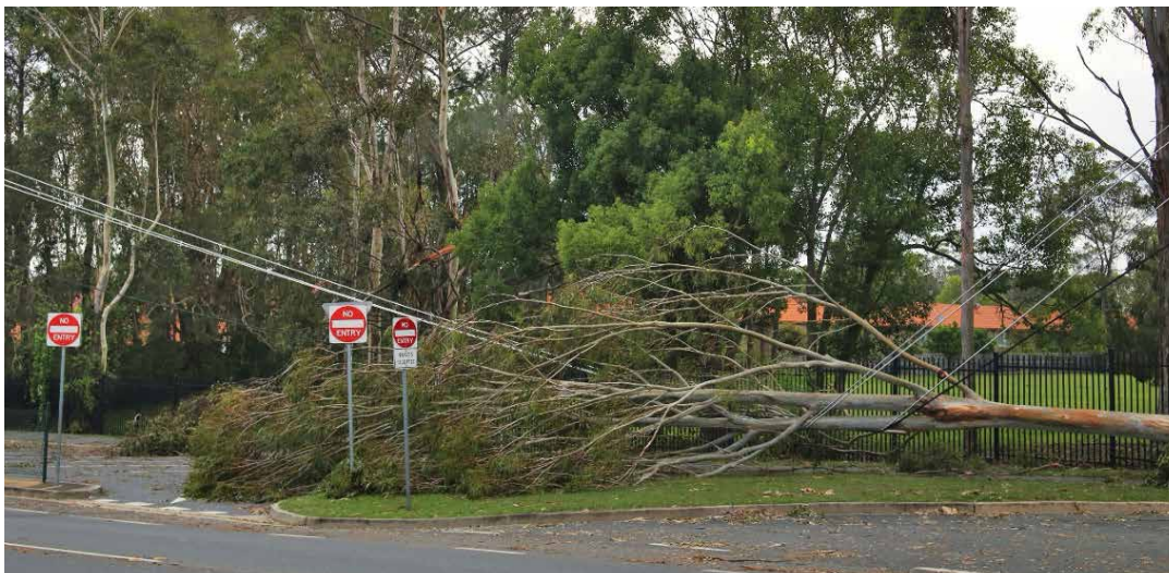
Figure 16. Powerlines damaged by fallen tree during severe storms on the Gold Coast.
