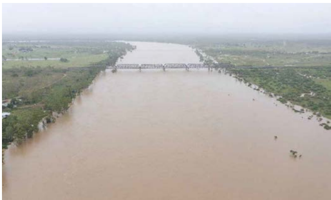
Figure 18. Flooding at Macrossan Bridge over the Burdekin River, near Charters Towers, Feb 2019
