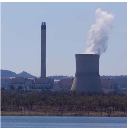
Figure 3. Callide coal fired power station. Source: Alamy
