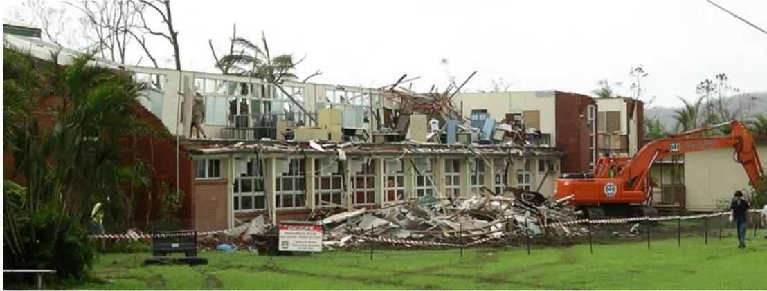
Figure 5 – Wind damage to roof structure and walls
