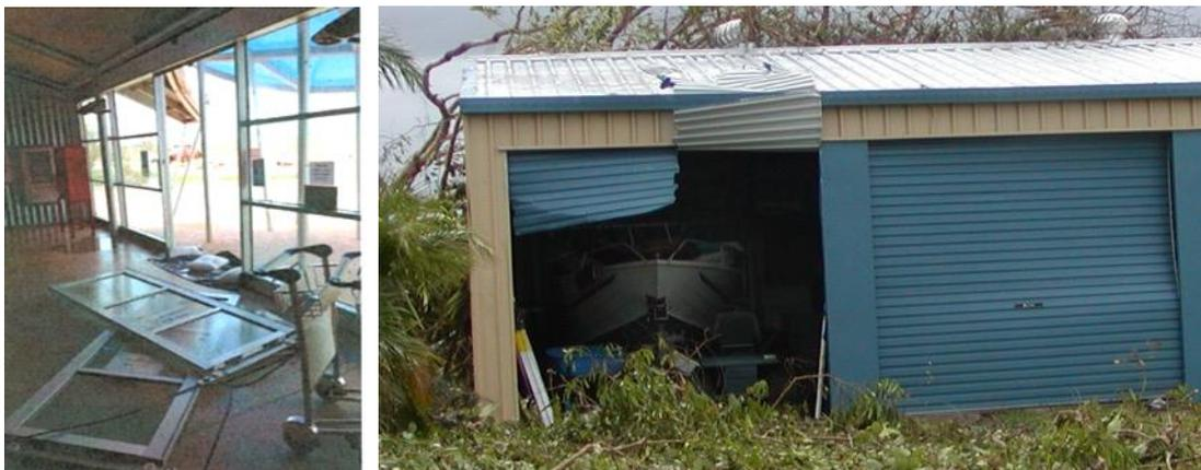
Figure 7 – Failure of automatic sliding doors and roller doors
