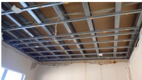
Figure 8 – Example of water damage to lower floor ceilings
