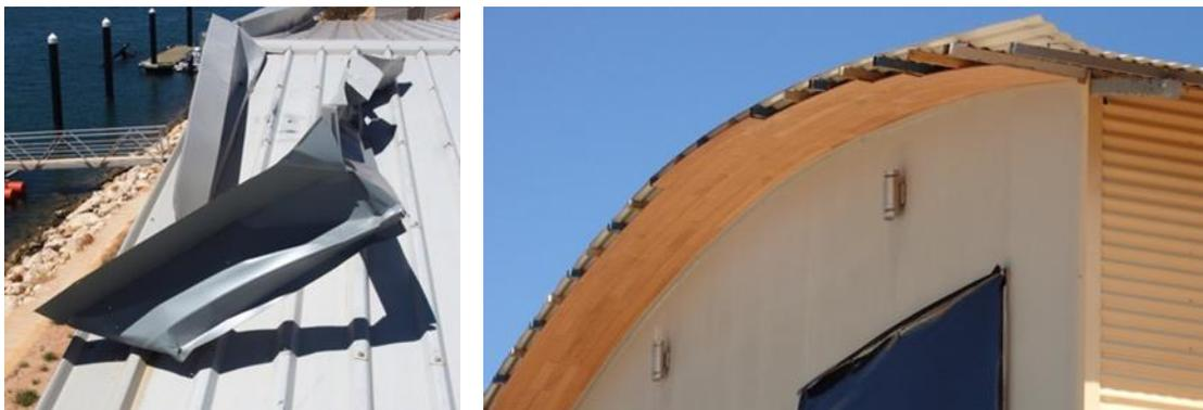
Figure 6 – Wind damage to flashings
